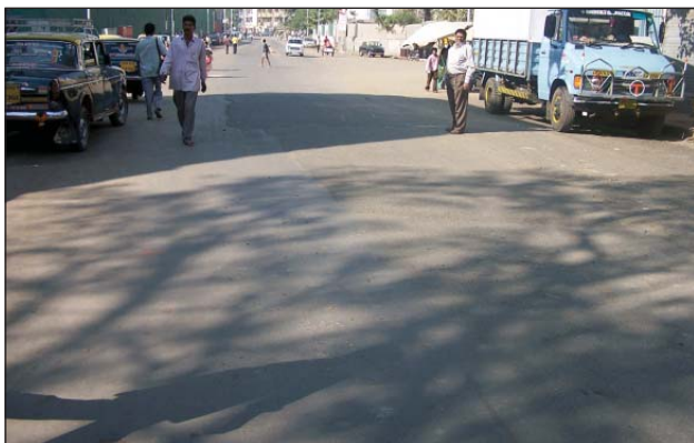
View of the road – 7 days after completion
