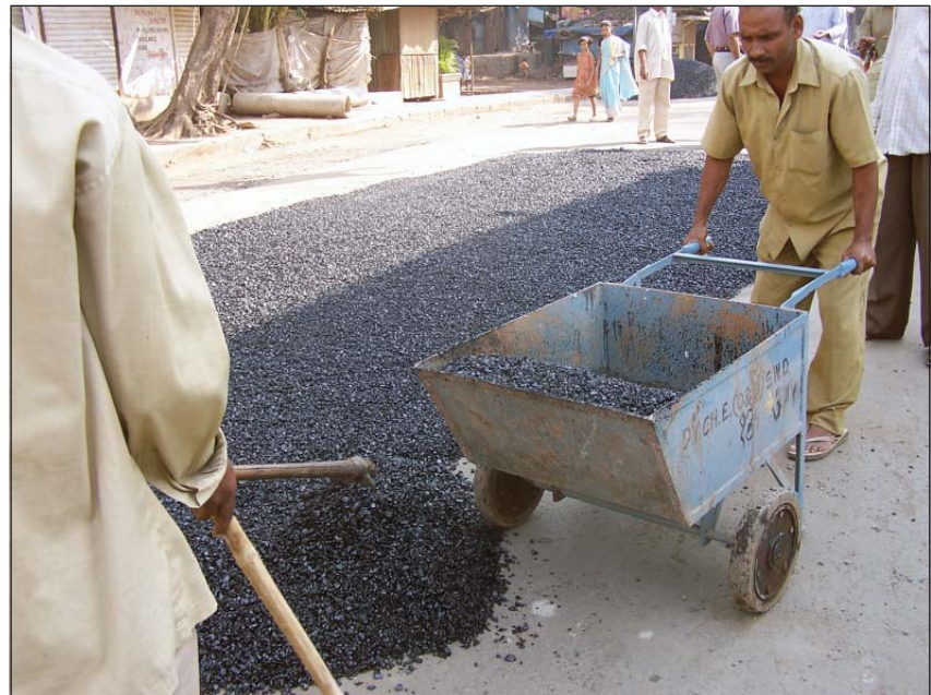
Tar road laying in progress
