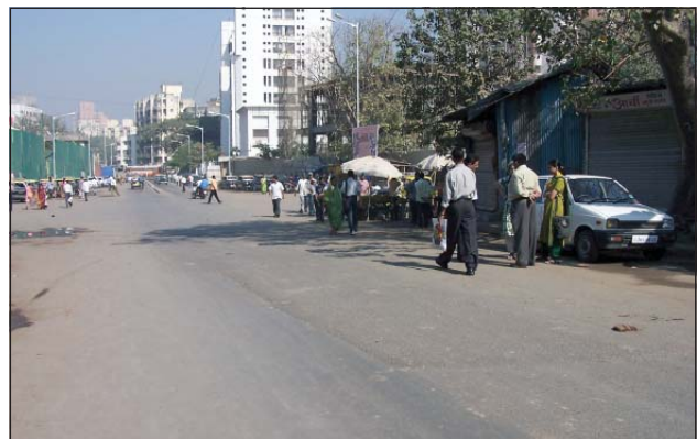
View of the road – 2 months after completion
