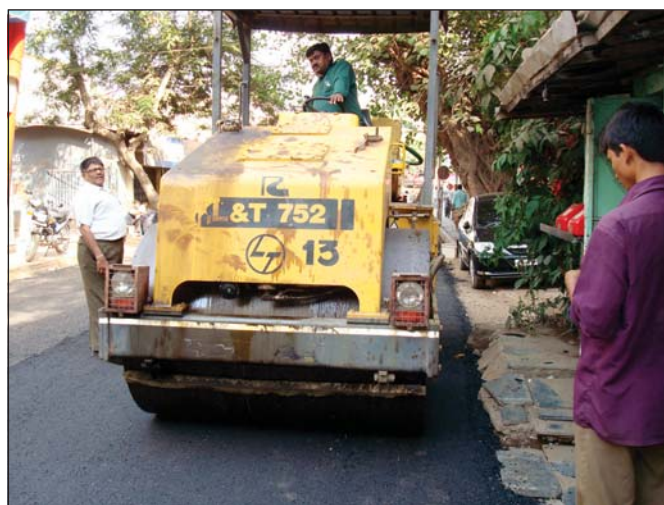
Construction of Tar Road using Plastics Waste in Mumbai.
