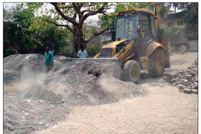
Ingredients being mixed with aggregate
