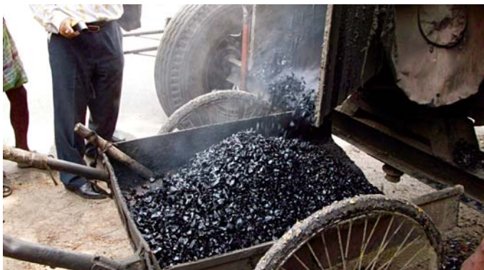
Step 4 : Hot mix discharge - ready for road laying
