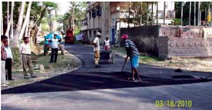
Seal coat being laid
