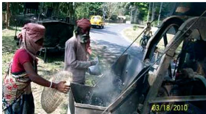
Plastics waste being spread over aggregates
