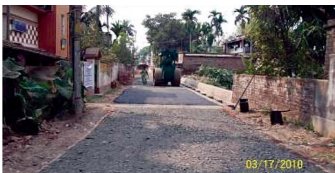
Road laying using plastics waste under progress
