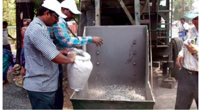
Step :1 Mixing of shredded plastics waste with aggregate
