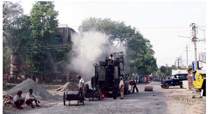
Step 3 : Hot Bitumen being charged
