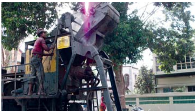
Step 2 : Aggregates mixed with plastics waste being charged into hot mix chamber
