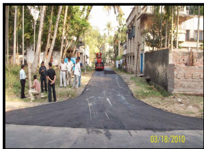
Completed road with seal coat. Ashok Nagar - Kalyangarh Municipality takes initiatives in this road construction using waste plastics for environment protection
