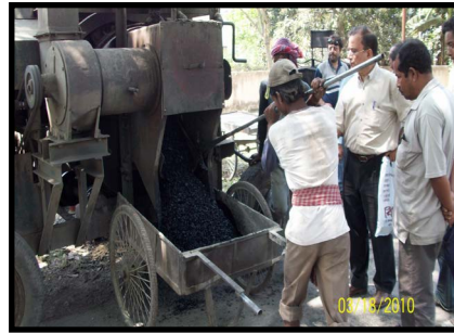
Blend is discharged at right temperature condition
