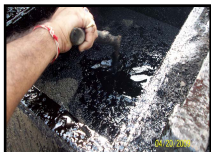
Mixing With Bitumen
