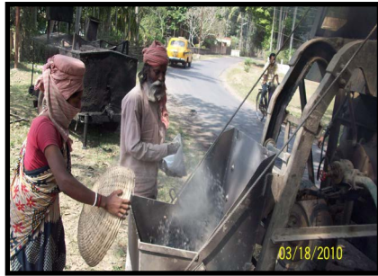
Road workers are mixing plastics waste with aggregates
