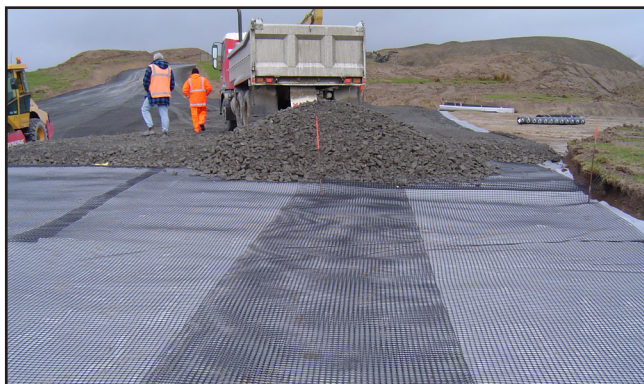
Reinforcement of road with Geotextile
