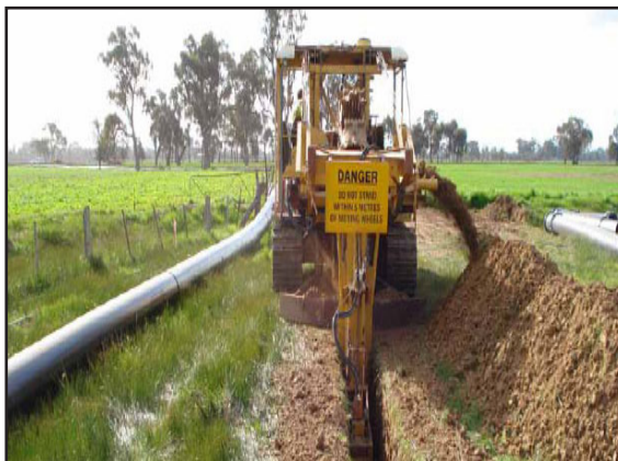
Trenching with pipe
