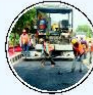
Work underway at site
