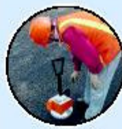
Depth of relayed stretch being checked
