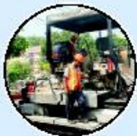
A road being paved with recycling technology
